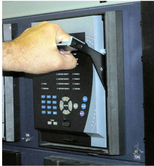
FIGURE 3-6: Rotate handle to stop position
