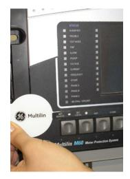
4. Slide the new user-programmable pushbutton label inside the pocket until the text is properly aligned with the
