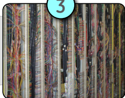
Thousands of individual copper wires from switchyard
