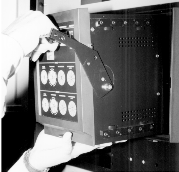
FIGURE 2-6: Relay Insertion
