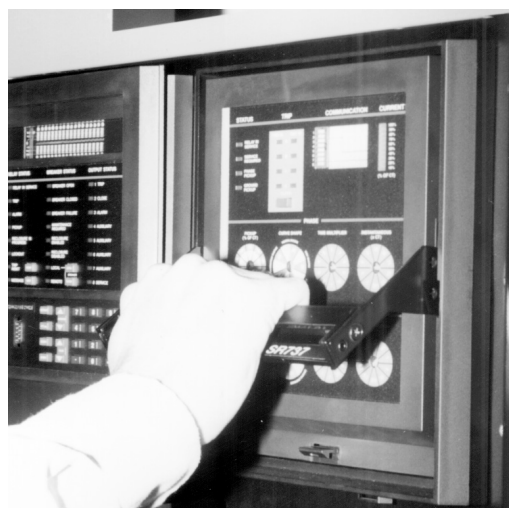
Press latch and pull to disengage handle
