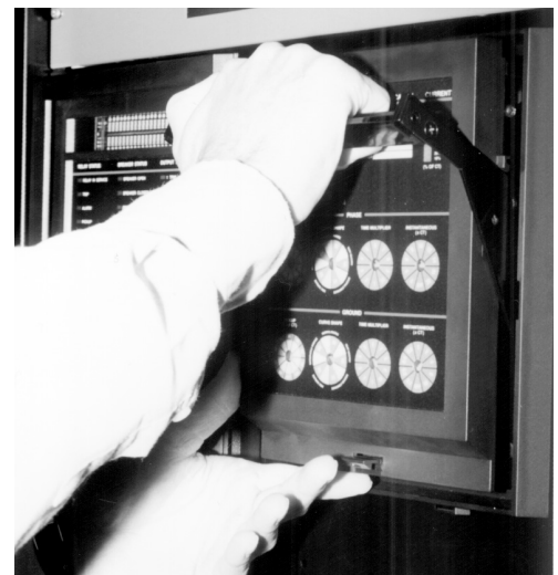
Rotate handle to vertical stop position and pull to withdraw
